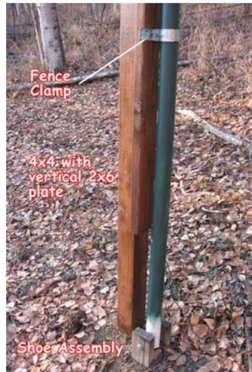
wanted to use a 2-inch U-bolt assembly to add stability. Unfortunately, the 4 x 4 is not wide enough, so it required a lag-bolted, four-foot 2 x 6 vertical extension to the 4 x 4 to provide the additional width. Once the pole is in position, a couple of strands of guy wire will run from the top of the mast to the same eye bolts used to guy the platform mast.
